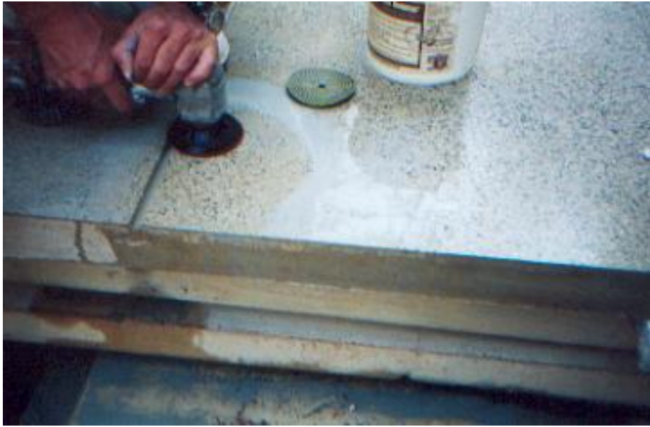
Grinding to produce a polished finish
