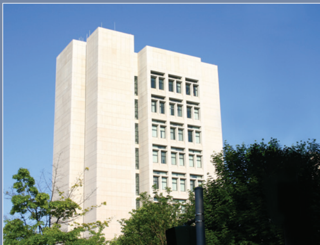
Westchester County Courthouse - Largest GFRC reclad in the US at the time: 220,000 square feet Westchester County, New York
