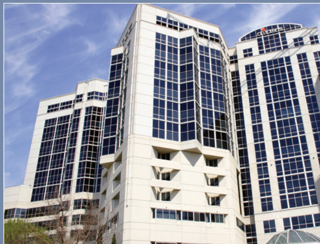
Children's Medical Center - Levels 7-12 Vertical Addition Dallas, Texas
