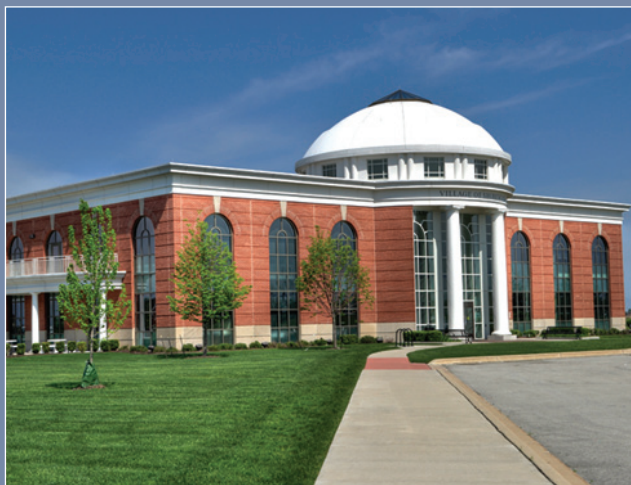
GFRC Dome - Shorewood Village Hall Shorewood, Illinois
