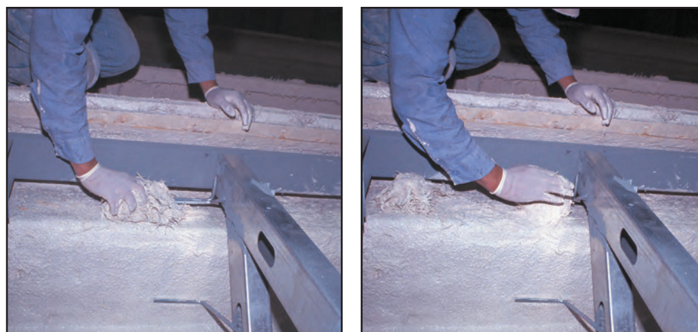
FIGURE 28.57 Making a bonding pad (also see Figures 28.52 and 28.53).
