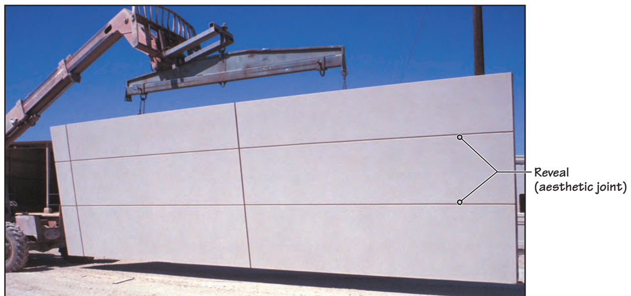
FIGURE 28.51 (a) The front face of a large GFRC panel after light abrasive blasting. It is being lifted for storage in the fabricator's shed.
