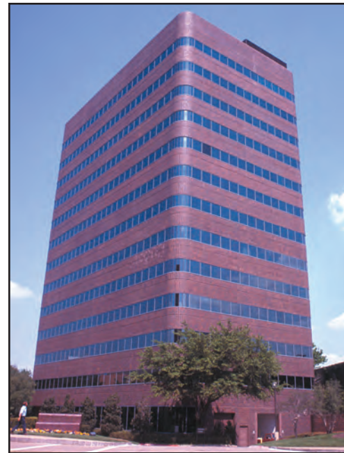
FIGURE 28.24 A building with brick veneer spandrels and ribbon windows.
