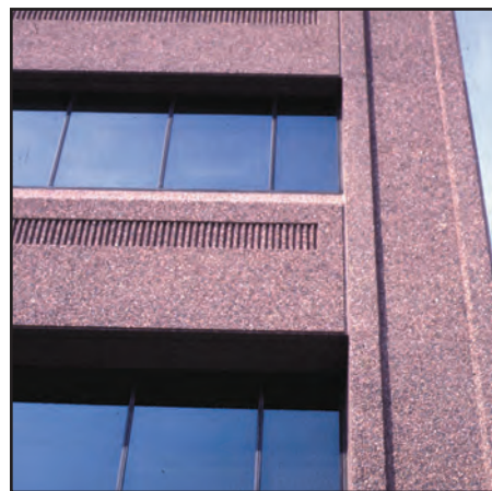
FIGURE 28.39 (c) Panel with an exposed aggregate finish.
