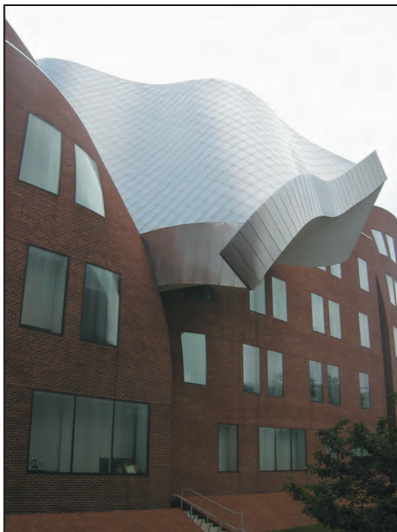
FIGURE 28.36 Warped brick veneer used in Frank Gehry's Peter B. Lewis Building, Cleveland, Ohio. (Photo courtesy of Doug Guth)
