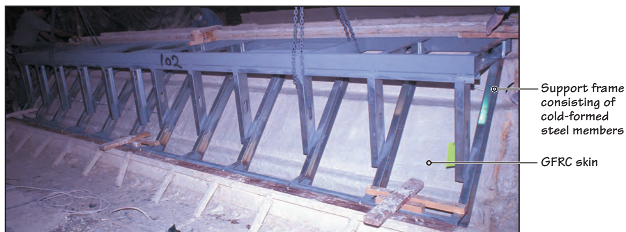
FIGURE 28.56 After spraying and consolidating the mix for the GFRC skin on the mold, a cold-formed steel supporting frame is placed against the mold and bonding pads are formed.
