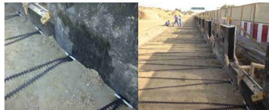
Aslan 600 Dowels as shear connector in MSE Retaining Walls.
