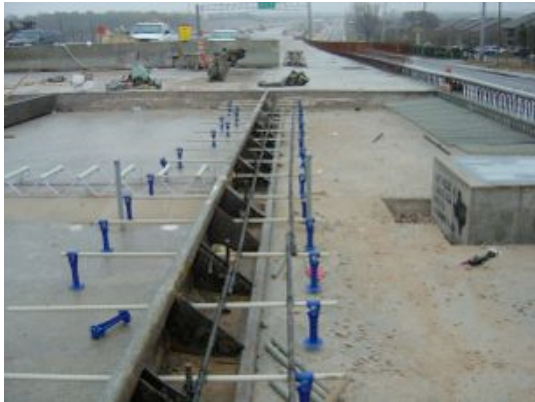
Aslan 100 GFRP Rebar is often used as “Tie Bars” in longitudinal joints.
