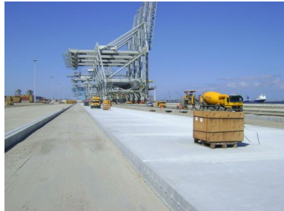
Section of Continuous Paving completed with Dowel Bar Insertion Machine
