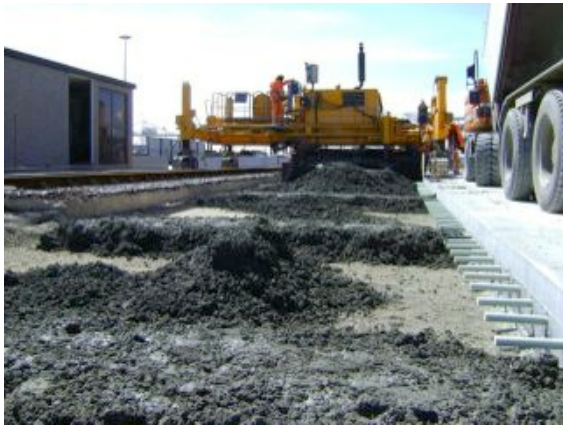
Drilled and Doweled GFRP Bars and Segmental Paving over Basket assemblies
