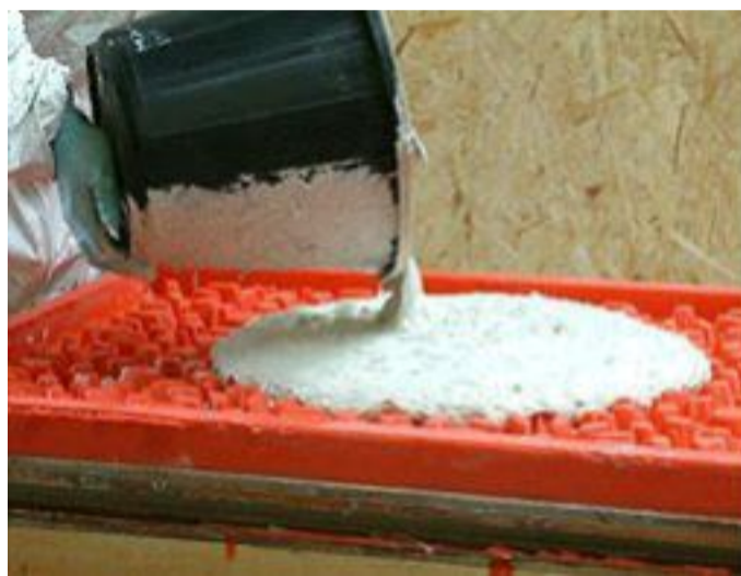
Premix GFRC pouring into moulds
